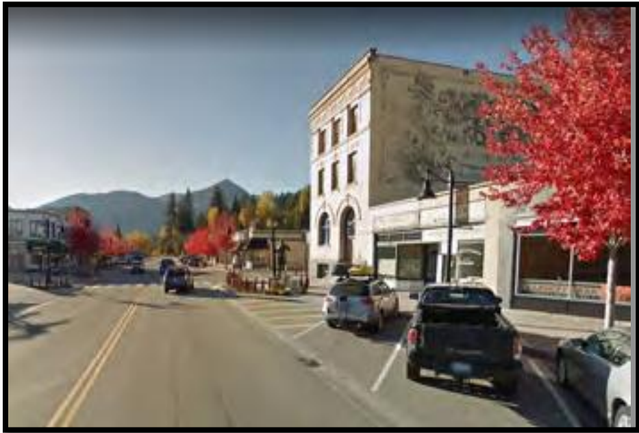
North side of Columbia Ave at Washington St.
